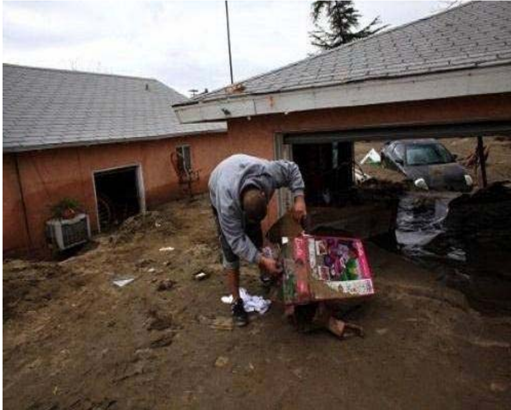
A mudslide severely damages a home and garage in southern California
