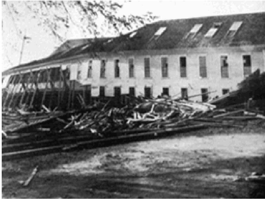
September 22, 1938, Bristol, RI. Damage to a building in Bristol. This storm traveled 600 miles in 12 hours, surprising Southern New England and causing widespread destruction. Photo courtesy of NOAA.
