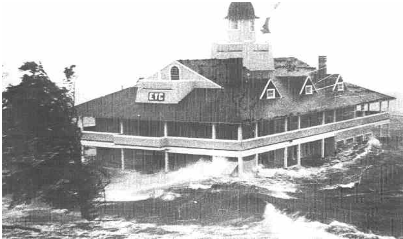
The Edgewood Yacht Club in Rhode Island is submerged by Hurricane Carol's storm surge in 1954. (Photo C. Flagg).
