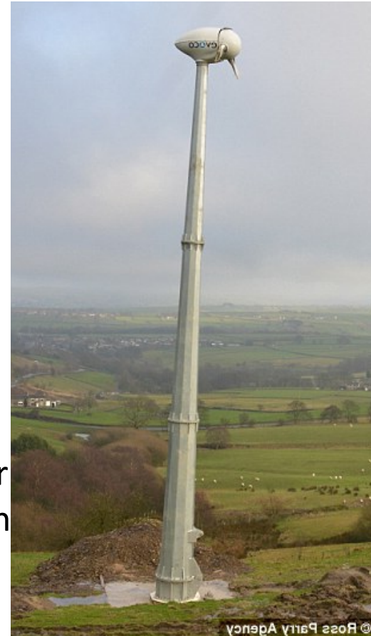
Scotland wind damage
